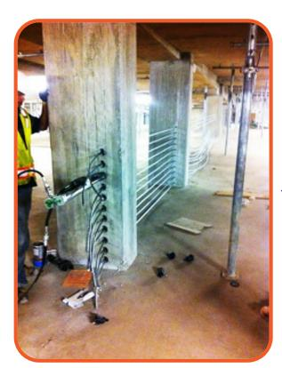
Tension cable with a calibrated PT Jack to the required force, extend the piston an additional 3/8" to anticipate wedge set then release (elongation recording is not useful or required)
