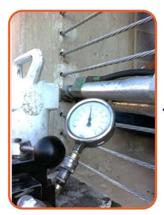
Feed cable from the stressing side to the opposite end and perform the back seating to a minimum 28 Kips at the Dead End
