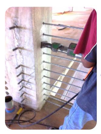
Perform the back seating to a minimum 28 Kips at the Live End (the 3/8" extra elongation are then lost as the wedge draws in to a permanent lock)
