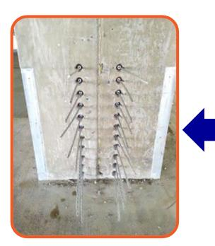
Trim tails inside the anchor pockets, patch pockets with non-shrink dry pack grout, touch-up jack gripper bites with cold galvanizing compound.
